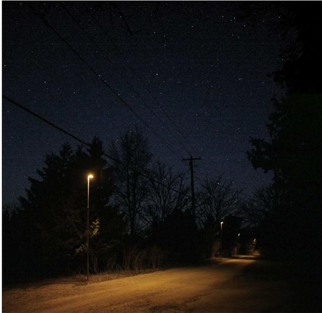
Low-impact lighting is used along an unpaved rural road (left). The amber spectrum helps preserve night vision, and sharp cut-off shielding minimizes glare and light trespass off the right-of-way. These images show the results for a 3-meter mounting height and 20 meter spacing.
